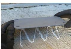
6. Position the plate in line with the markings.
