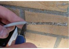
6. Carefully cut and remove the braided sheath.
