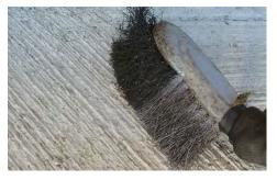
4. Any grease or silicon under the plate will prevent the adhesive from making a solid bonded connection so de-greasing the surfacing may be necessary.
