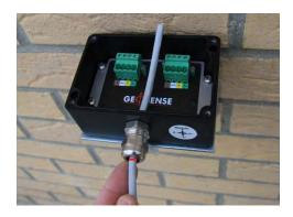
3. Draw the cable through the gland until the mark is clearly visible.
