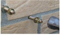
5. Remove any dust from the holes and insert the fixings.
