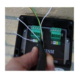
11. Carefully draw the wire back out of the gland until the braided section is just visible.
