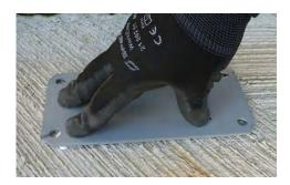
7. Press down firmly on the plate, and where necessary, hold it, or leave it in place, until the bonding agent has cured (set).
