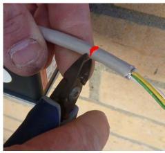
8. Remove the sheath to expose the braided shield.
