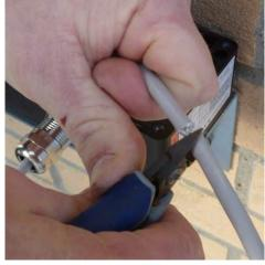
5. Remove the sheath to expose the braided shield.
