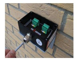
2. Insert the cable into the EMC cable gland and push it through until it reaches the back of the box. Mark the cable as shown.
