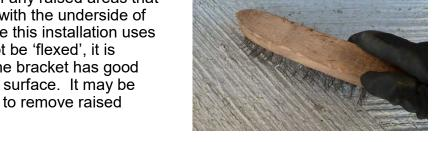
3. Clean the surface under the plate with a wire brush and remove any dust from both surfaces.
