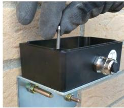
11. Using an 'Allen' key, secure the fixing screw.
