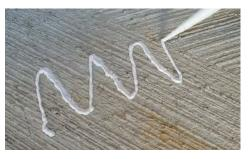
5. The selected adhesive should be applied in accordance with the manufacturers instructions. Ensure enough adhesive is applied to bridge any undulations and provide a good bonding surface.
