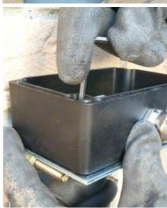
12. Locate the other sixing screw and tighten both screws to fix the box to the bracket securely.
