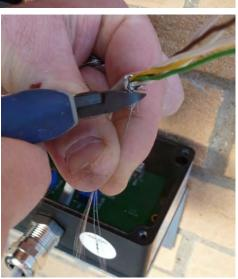
7. Measure 30mm back from the end of the sheath and carefully cut the sheath using either cutters or a sharp knife. Take care not to cut the braided shield.
