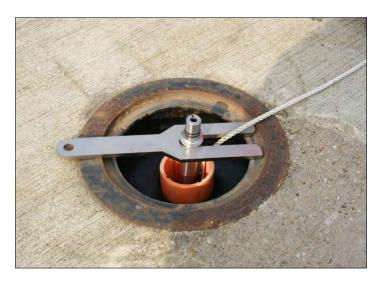
**STEP 11 -** identify the next IPI sensor to be installed and remove the **RED** plug from the connector
