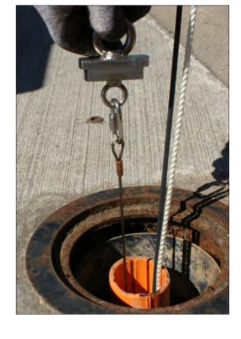
**STEP 20 -** once the top collar hanger rests on the top of the casing secure the support rope to its final location.
