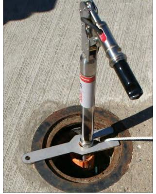
**STEP 11 -** Continue lowering the assembly until the installation fork rests on the top of the borehole
