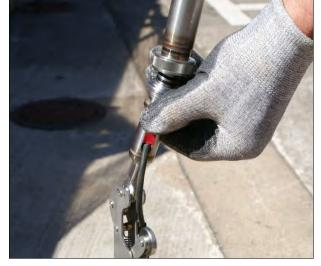
STEP 13 - Remove the top BLACK dust cap from the previously installed IPI sensor and carefully align the
