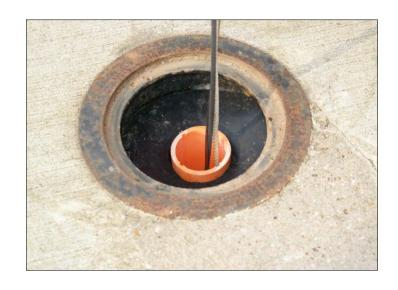
STEP 17 - identify the top IPI sensor and connect one end of the top support wire rope using the Rapid Link
