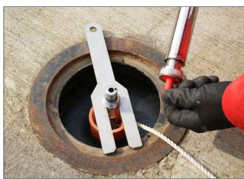
STEP 12 - align the two connections
