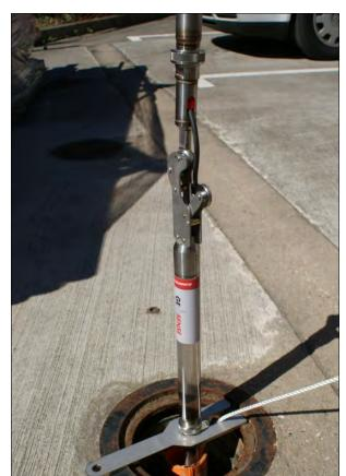
**STEP 15** - Raise the assembly a little and remove the installation fork
