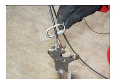
**STEP 15 -** lift to remove the installation fork and lower the assembly into the casing
