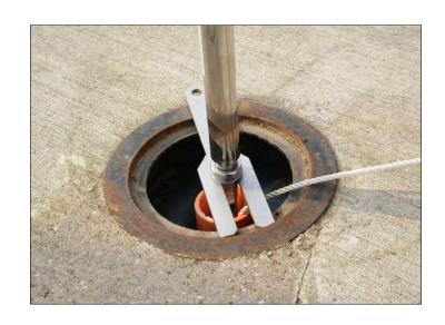
**STEP 14 -** connect the Rapid Link on one end of an intermediate wire rope support onto the top of the IPI sensor
