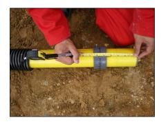
7. Place the magnet over the access tubing and screw the datum magnet in place with the provided Allen key.
