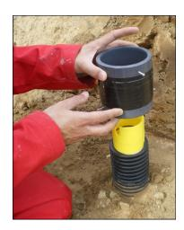
23. Screw the corrugated piping in place with the screws provided.
