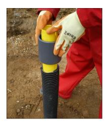
15. Attach coupling joint to corrugated piping with the screws provide.
