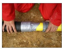
9. Install the casing into the borehole, with the datum magnet end of the access tubing going in first.
