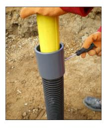
16. Place top cap on access tubing. This is to ensure that no fill enters the access tube.
