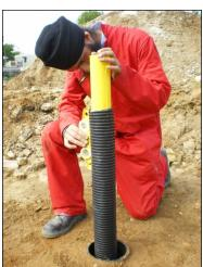
12. Fill borehole with bentonite pellets.
