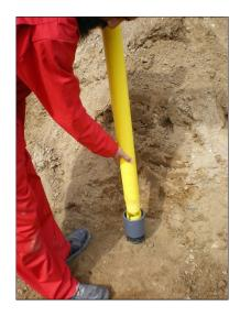
19. Place the next corrugated piping over the access tubing and into the coupler, ensuring that the corrugated piping is firmly in the coupler.
