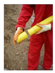
4. Insert the casing into the corrugated piping. Ensure the corrugated piping is taken above the end of the access tubing.
