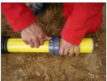
8. Duct tape around the corrugated piping and the access tube.
