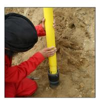
25. Place the next corrugated piping over the access tube and into the magnetic coupler, ensuring that the corrugated piping is firmly in the magnetic coupler.
